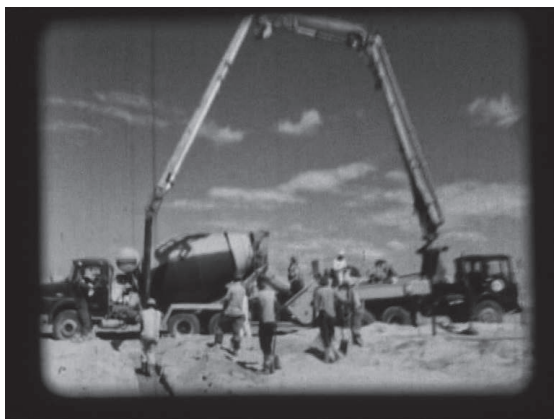
Fig. 3.9 Workers and house bases (2)
