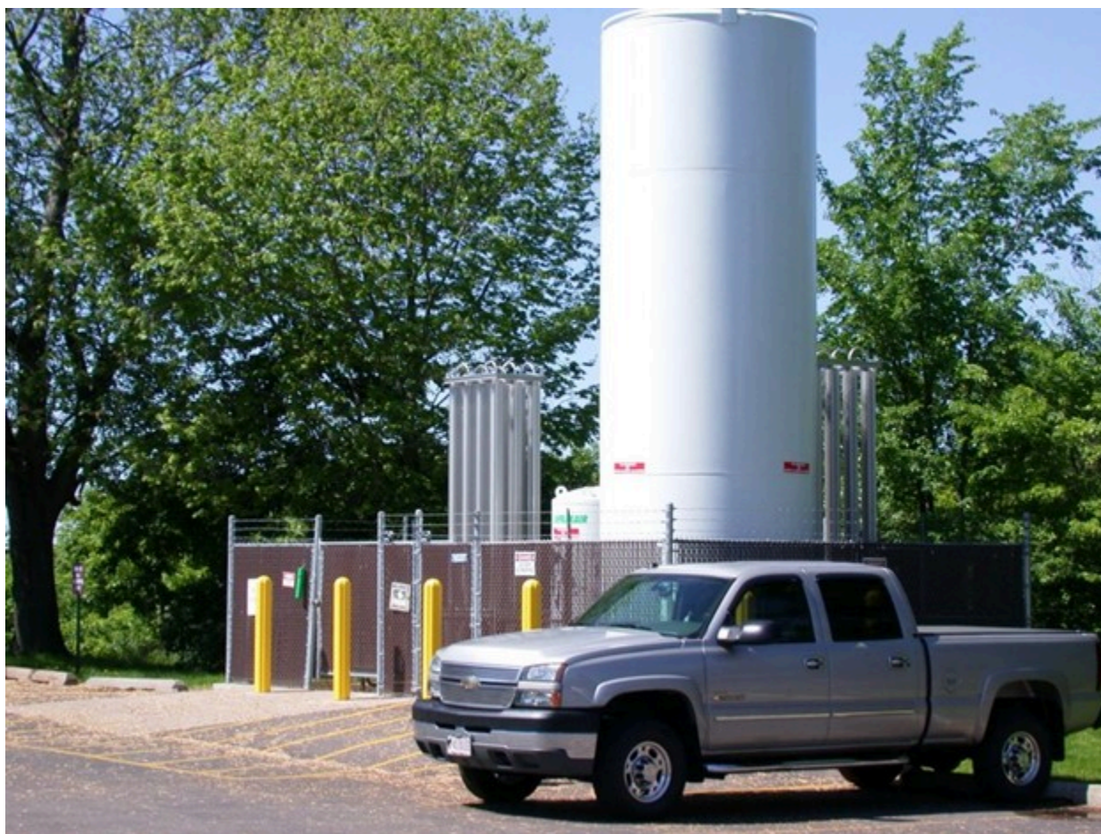
Figure 12. Liquid oxygen tanks outside of a hospital.
